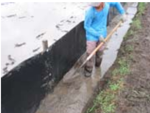
Building a Trap Barrier System.
